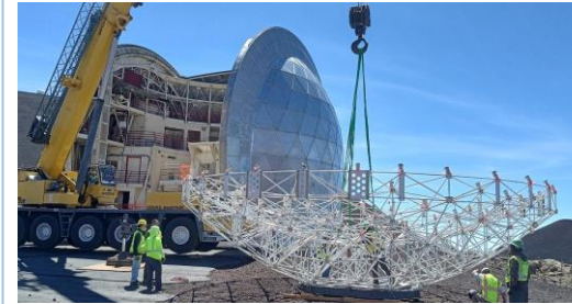
Decommission of CSO is ongoing and featured in local media.(Sep. 2023)
