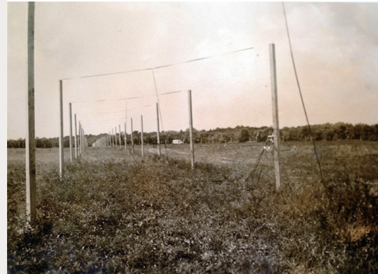
Figure 01: The antenna was designed by B. Y. Mills, an Australian radio astronomer, and Martin Ryle of England, who later won the Nobel Prize for aperture synthesis in interferometry. It was made of 66 pairs of wooden masts with wires strung across the tops of them. The total length of the wires used is said to have reached 8 km. The receiving equipment was mounted on an army surplus truck which was already on the site. Unfortunately, it has now been removed, neither the station nor the antenna remain. Credit: Carnegie Institution for Science Archives
