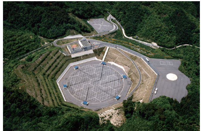
Figure 28: An array of 475 antennas arranged in a circular area 103 m in diameter. The MU Radar can not only transmit signals in phase to give direction, but also change the direction of the signals 2,500 times a second.
