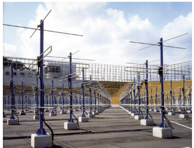
Figure 29: The crossed Yagi-Uda antennas arrayed on the ground; equipped with a small transmitter-receiver module, each one can transmit and receive radio signals. Although the MU Radar was originally intended to observe the spatial structure of high-altitude winds and atmospheric turbulence, it can also observe meteors because meteors (or more correctly their head plasma) in the atmosphere reflect radio waves with frequencies that the MU Radar covers.
