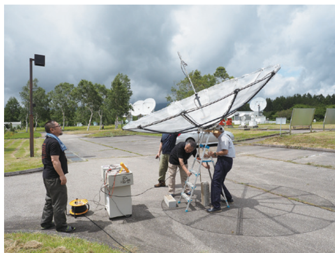
05 The parabolic antenna has been completed!
