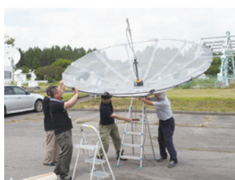
02 Diligent work to stack two sheets of wire mesh and binding them together to the PVC pipe frame with thin wires.
