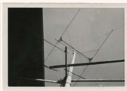
03 (Left) A 6 element Yagi-Uda antenna for 15 m wavelengths (constructed August 1962); (Right) A 2 element loop antenna for 15 m wavelengths (constructed October 1962); after a typhoon struck, I had to construct a new antenna after only two months.
