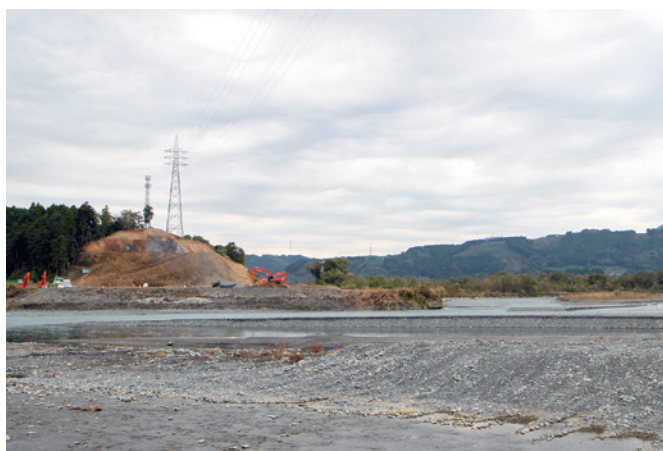
11 A photograph of the river channel widening work taken from the bank opposite of Mt. Ushio. The part jutting out into the river is being chipped away leaving effectively level ground.
