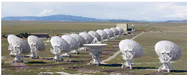
Figure 13: The Karl Jansky VLA (Very Large Array), shown here during observations, is composed of 27 antennas with diameters of 25 m each, arranged in a "Y" pattern."
