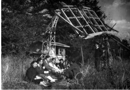
Figure 01: 1949, the beginning of 200 MHz intensity observations. Eight dipole antennas were arrayed on the approximately 5 m x 2.5 m wooden frame. It seems the equatorial mount was repurposed from one used in an optical telescope.
