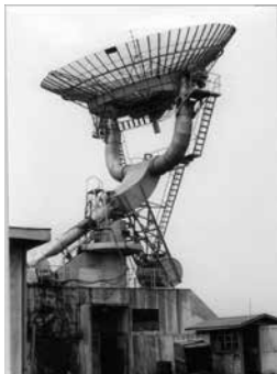
Figure 03: 1953, the start of 3 GHz observations using a 10-m parabolic antenna in Mitaka (refer to the front page as well).
