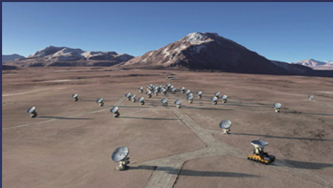
ALMA is an interferometer capable of repositioning each antenna for observations.
