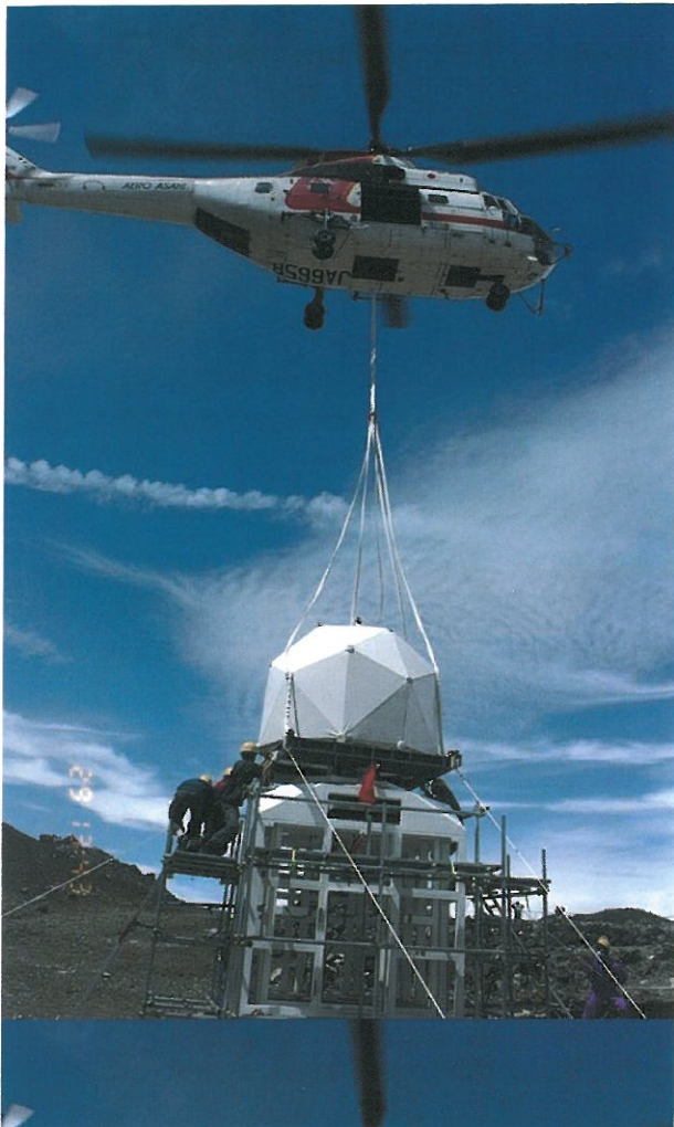
Figure3 Installation of the Mt Fuji submm Telescope by a helicopter
