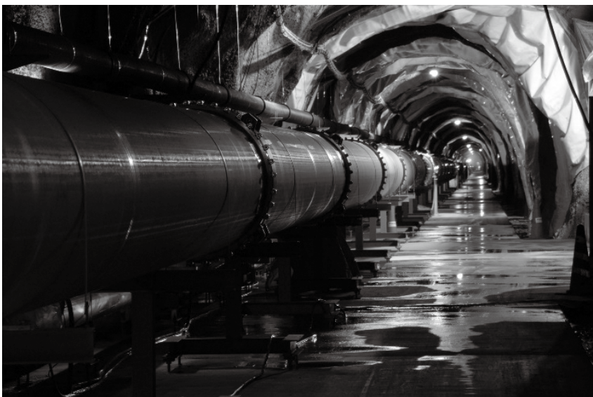
Figure 1: KAGRA construction progress: while the arm ducts are installed at Kamioka, the first full prototype of the vibration isolation system is tested in one of the TAMA vacuum chamber at Mitaka.
