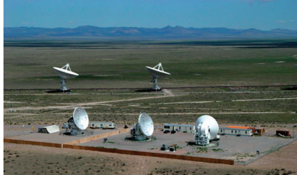
Figure 1: Three ALMA prototype 12-m antennas (front) at the NRAO VLA site. The NAOJ antenna (left) was used for the measurements. Two 25-m antennas (back) are element antennas of the VLA.
