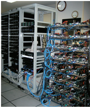
Figure 1: Photo of our clusters. Left side two 19-inch racks hold 16 nodes, where each node consists of an Opteron 250 CPU and a GRAPE-7. The aluminum rack in the right side holds other 16 nodes, where each node consists of two Opteron 244 CPUs without any GRAPEs. Gateway, file server, network switches are installed between the two clusters.
