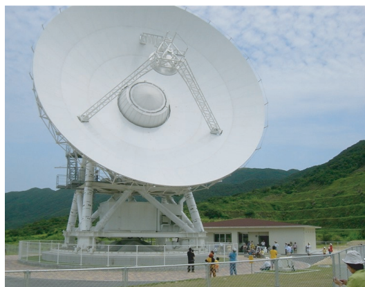
Figure 1: Top : 20 m antenna under construction with 200 ton crane (Autumn, 2001), bottom: Visitors looking at the moving telescope in the openhouse held in the day after the Opening Ceremony
